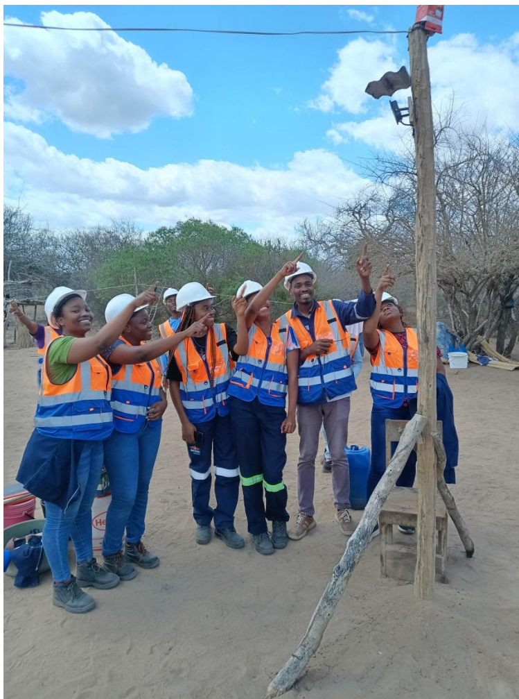
Photo: Photocell with its lamp successfully mounted.
