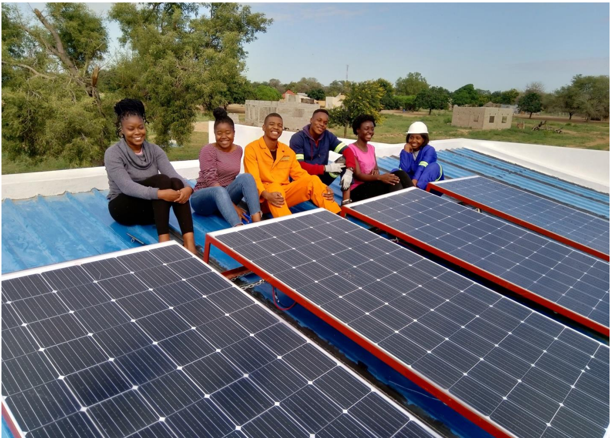
Figure: Happy End, Photovoltaic system successfully installed.
