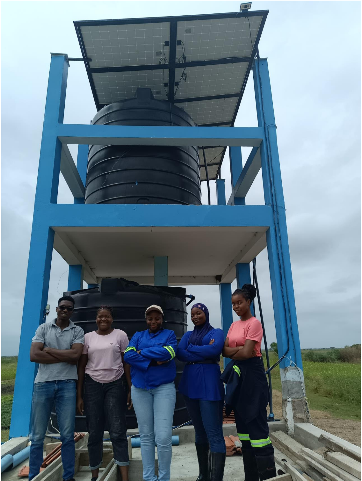
Photo: Trainees parade alongside a photovoltaic water pumping system during a training course on the topic: Assembly and Operation of a Residential Electrical Installation and an Isolated Photovoltaic System.
