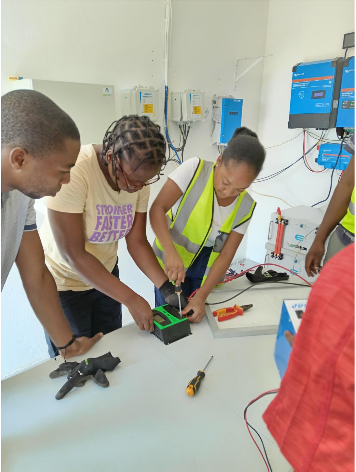
Photo: Women during the assembly of a photovoltaic system.
