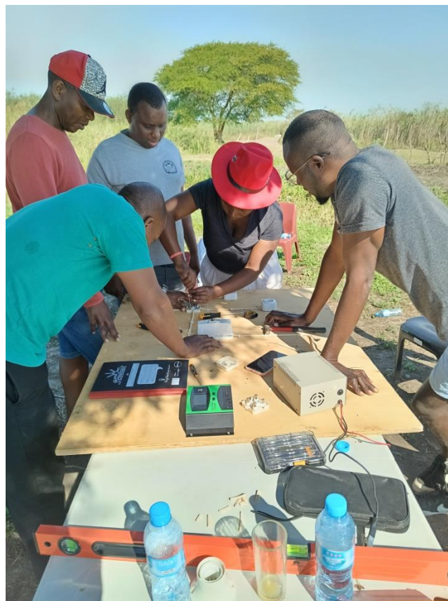
Figure: A Woman during the installation of a photovoltaic system
