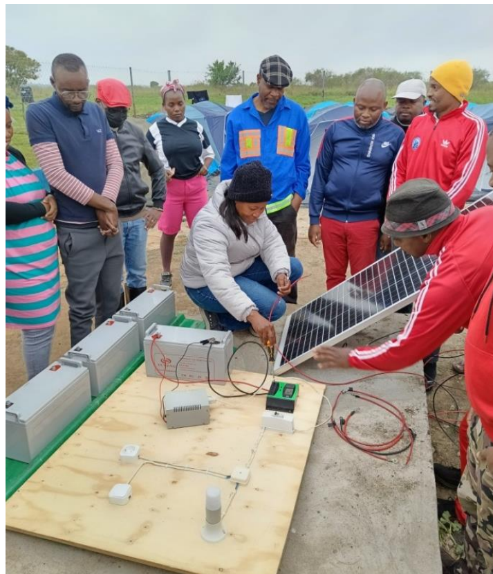
Figure: A Woman during the installation of a photovoltaic system
